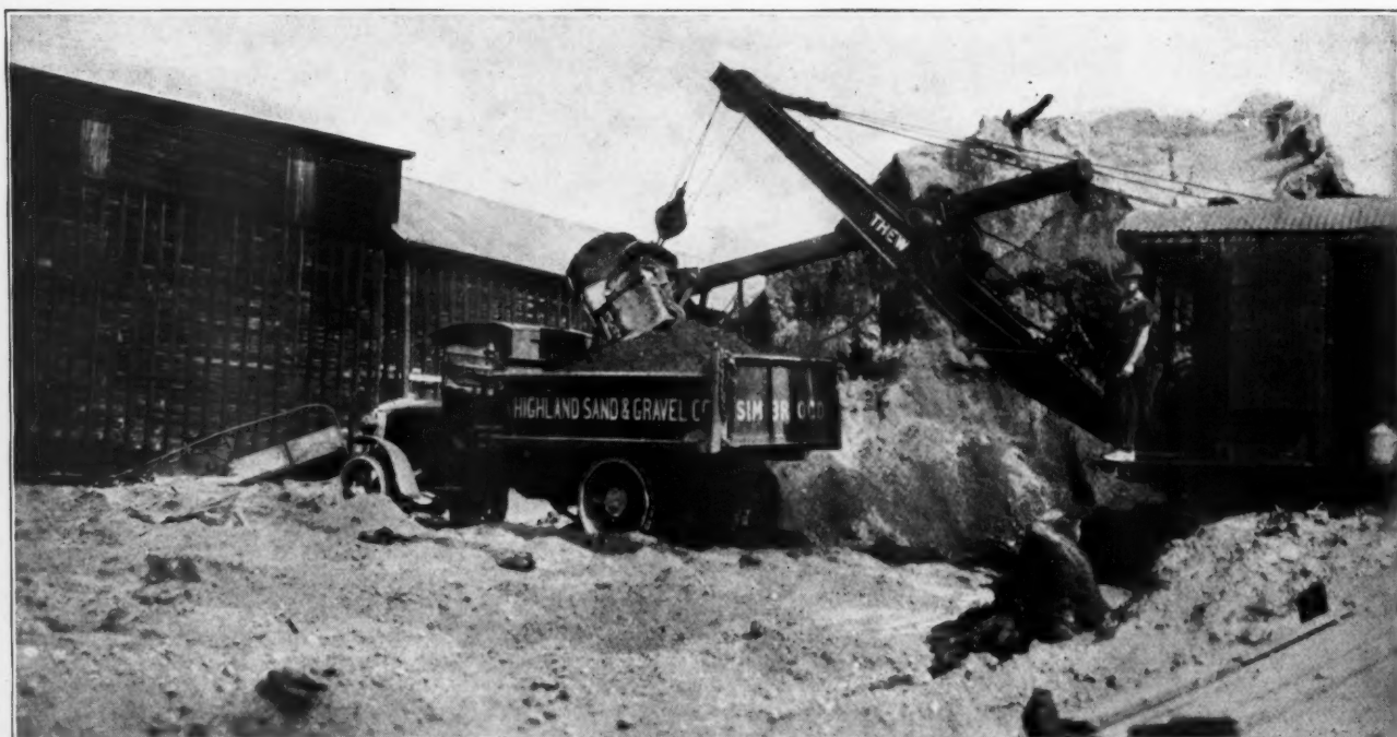
Gasoline Shovel Loading Overburden into Truck
